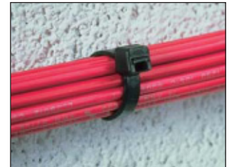
4. Install wires or cable.
