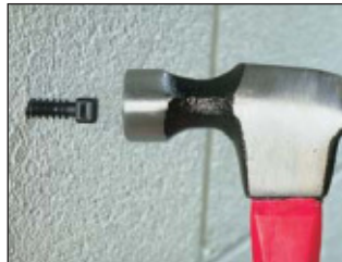
2. Hammer mount into hole.
