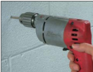
1. Drill hole using correct size bit.
