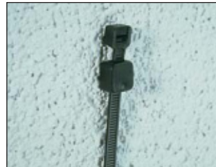
3. Place cable tie through mount.
